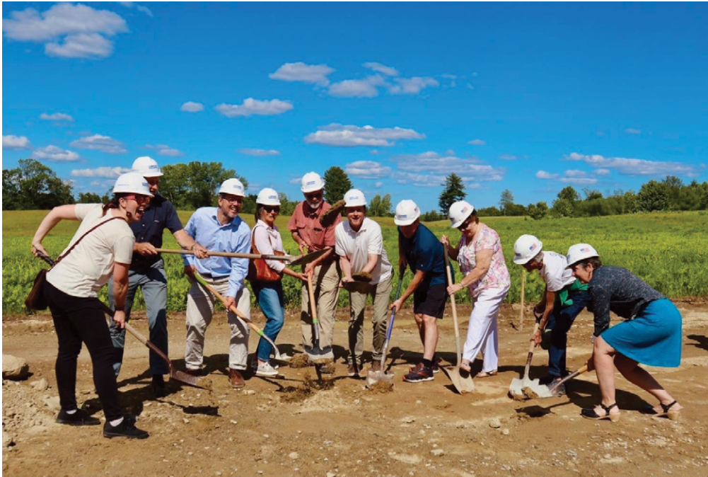
The shovels go in the dirt at the Mathey Center groundbreaking ceremony.
