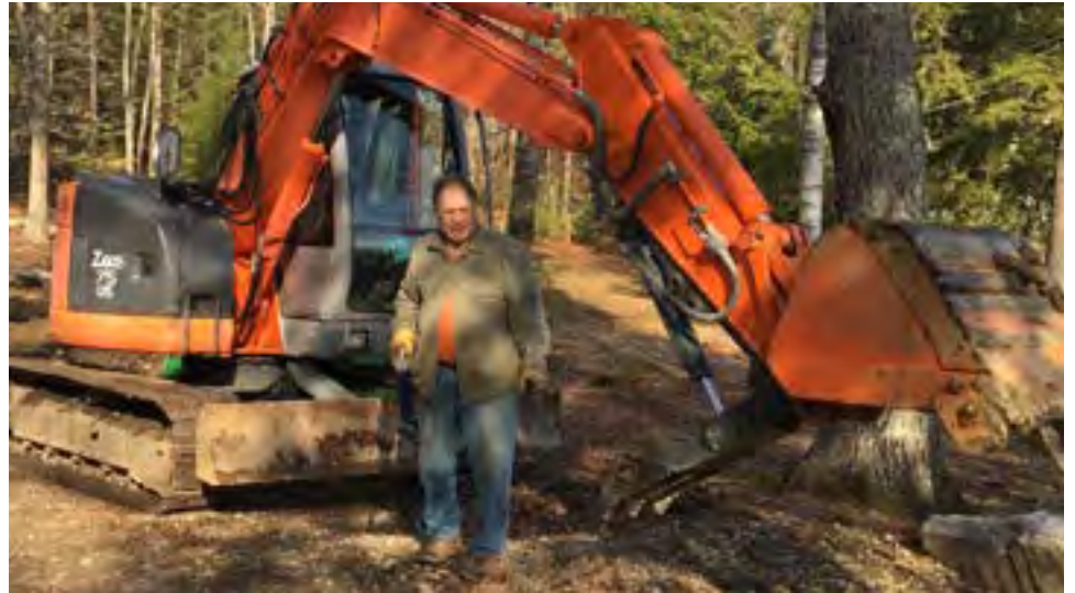
Carl and his excavator. COURTESY PHOTO
