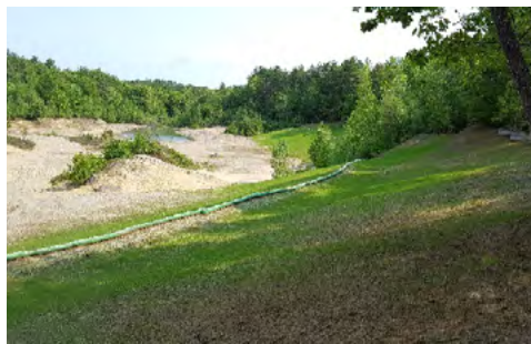
Above: April 2, 2019 – During – Reducing the slope. PHOTO: JENNIFER PRIBBLE
